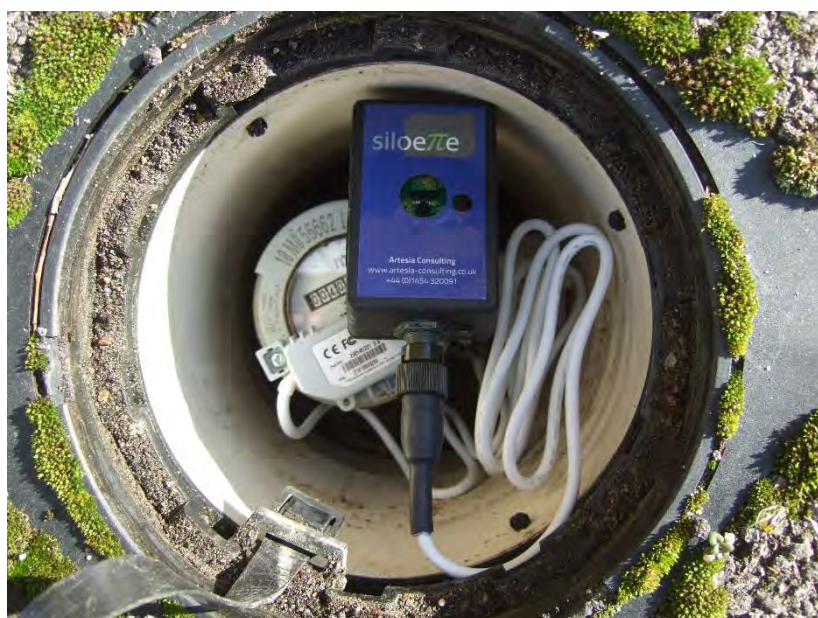
Figure 3 Siloette logger installed in a boundary box
